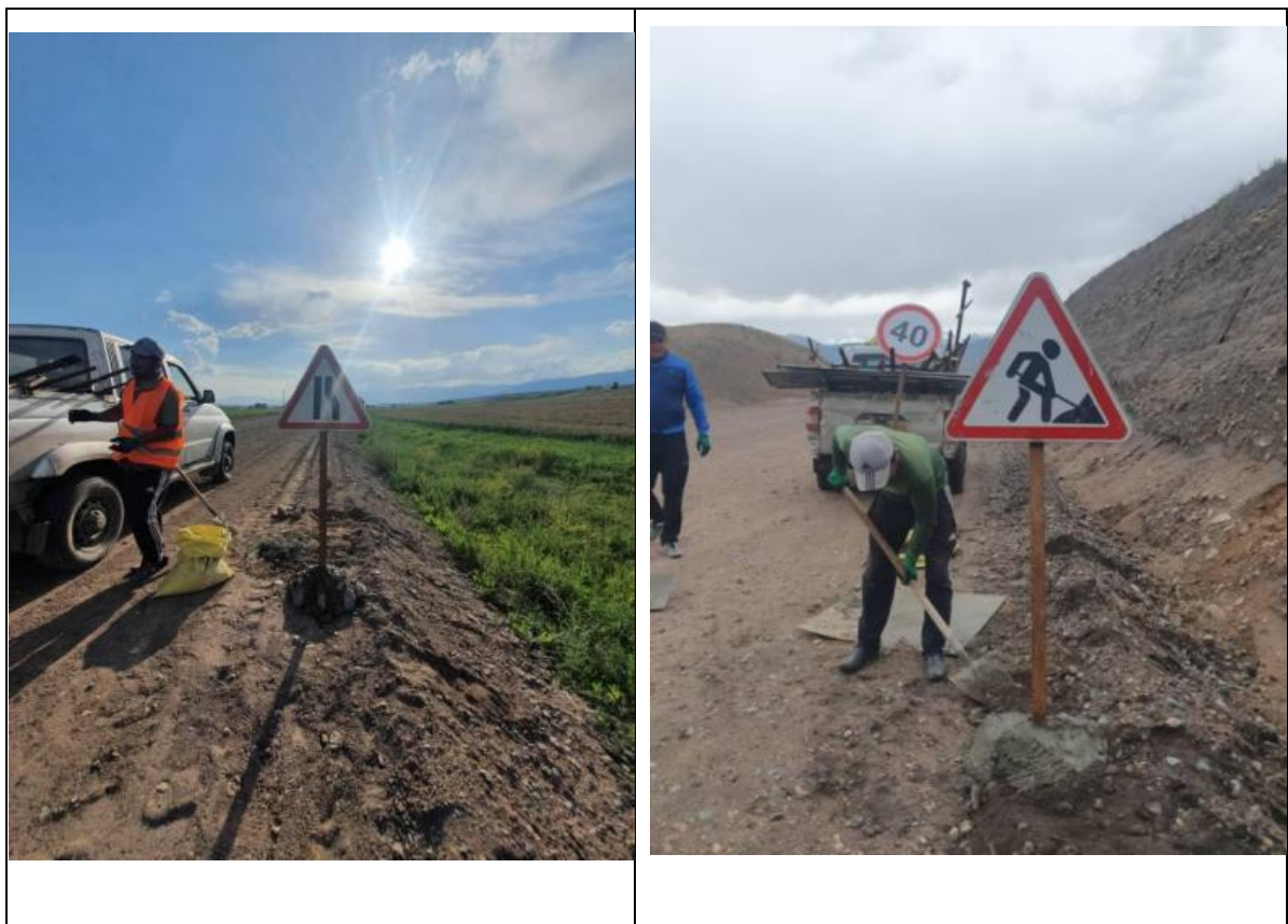
Figure 3 Temporary road signs installation.
