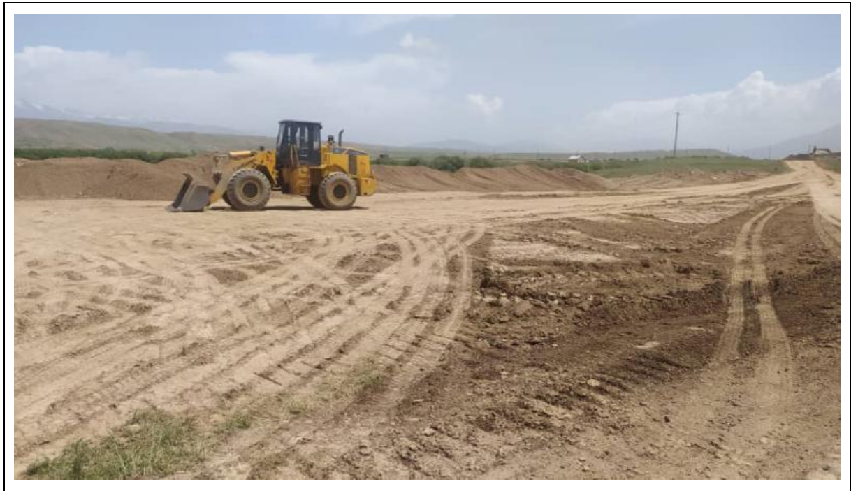
Figure 8 Quarry development (km.140+990).
