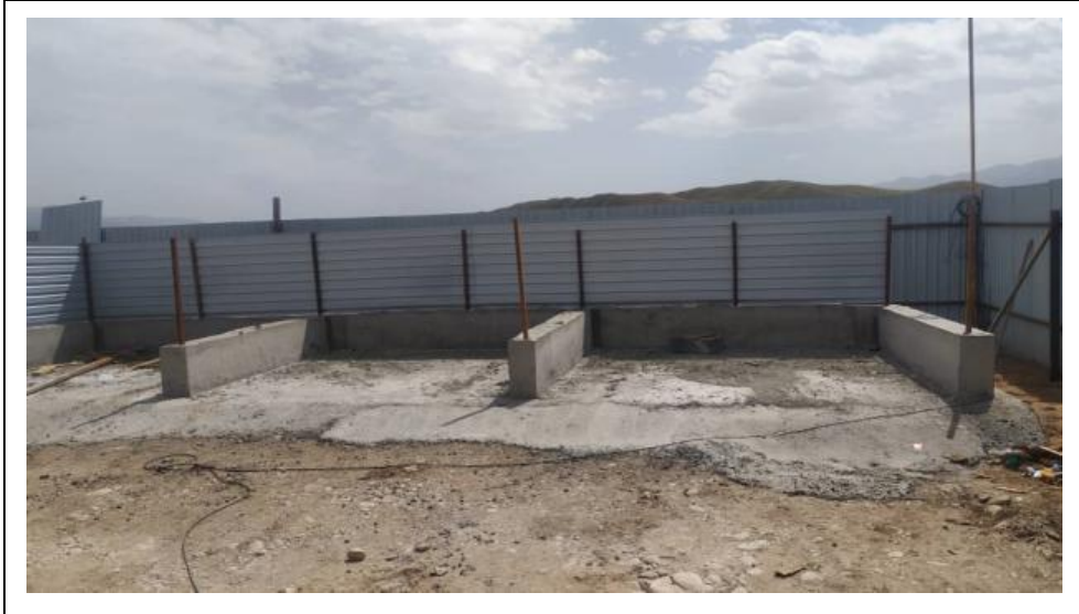
Figure 20 Preparation of a waste site at the camp territory.
