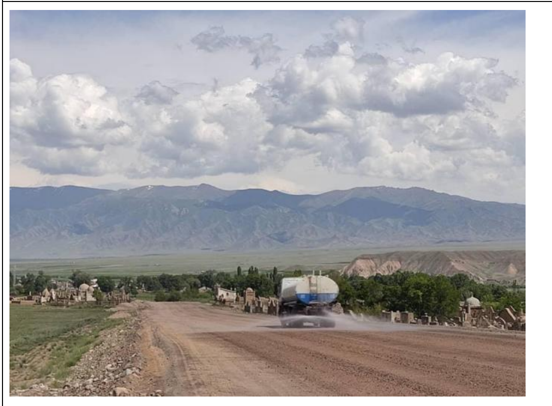
Figure 7 Dust suppression on roads.
